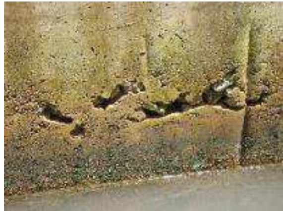
Void caused by insufficient compaction
