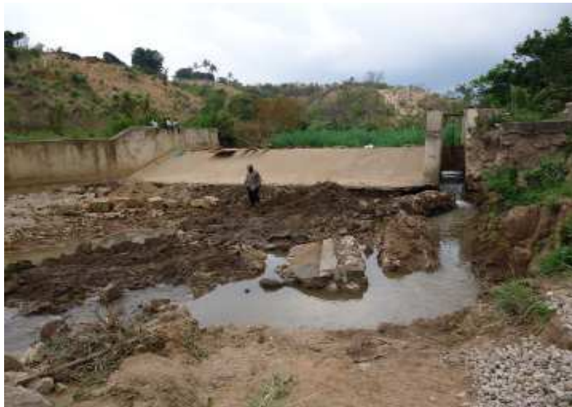
Left side wall collapsed by scouring / erosion occurred by flood water. (View from downstream)
