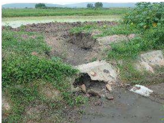
Collapsed canals by overflowing of floods
