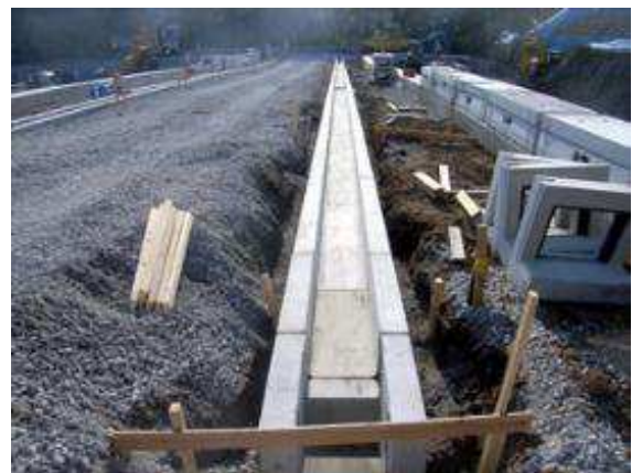
Keeping materials tidy up
