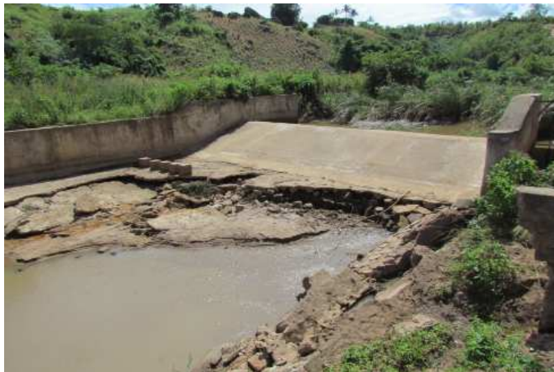
Base concrete washed away and hydraulic jump broken by piping and flood power.
