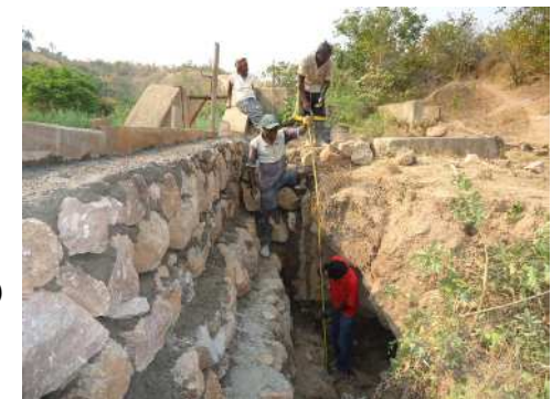
Increased depth of the embedment to 1.2m from the base of downstream apron.
