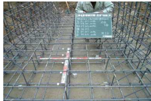
Finishing reinforcing bar setting
