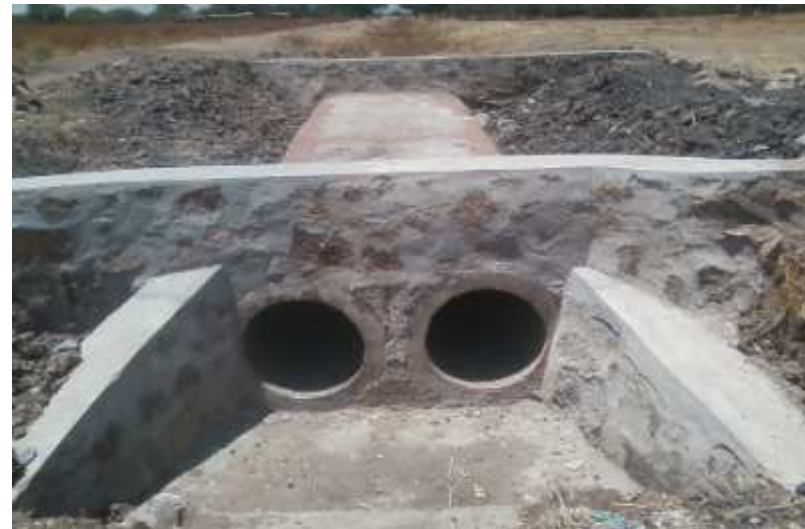
Two concrete pipes will allow more water to pass through and prevent overtopping. Moreover, the wing walls which prevent scouring hence no seepage were installed at the entrance of the pipes.
