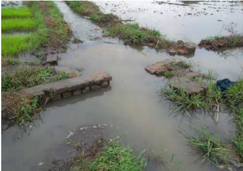
Collapsed division box is selected as main problem after Participatory Diagnostic Study.
