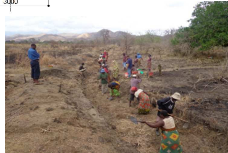
Removal work of sand on catch drain with farmers' contribution.
