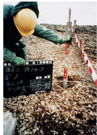
Finishing backfilling
