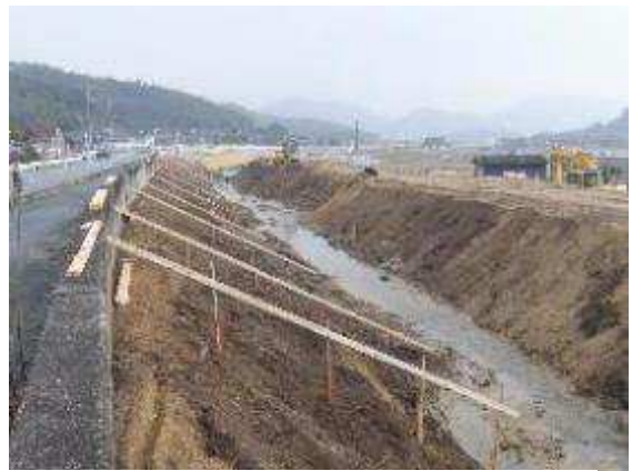
Setting the guide bar for side slope arrangement
