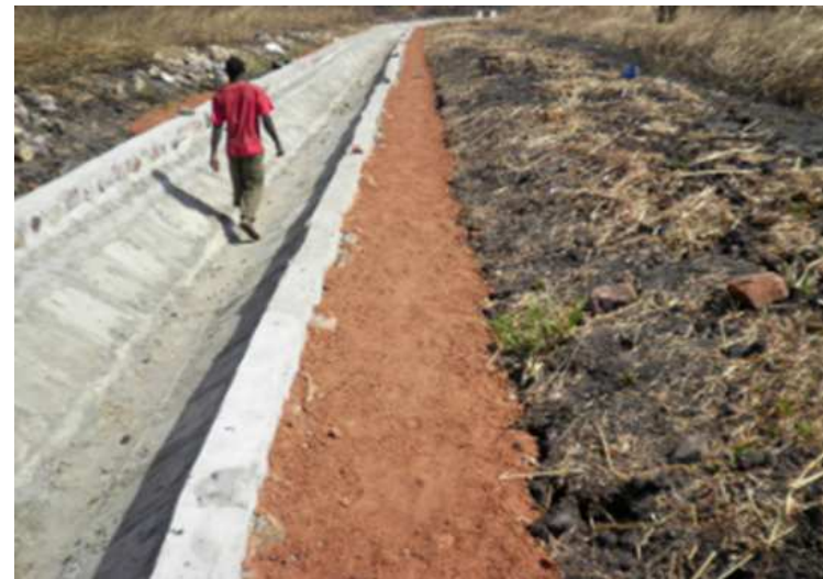
Backfilling was imported and compacted using good type of soil.
