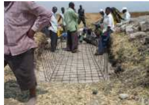
Reinforcing bar setting on the well compacted foundation.
