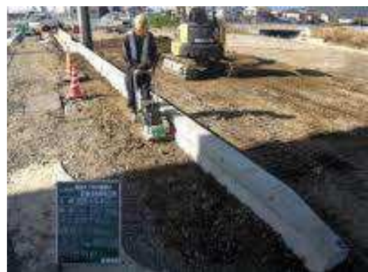
Compaction at the road construction
