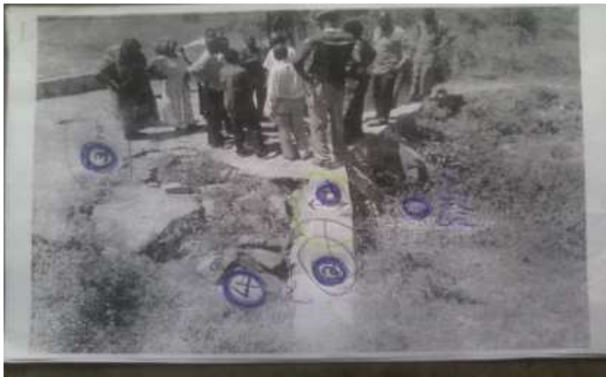
Vented drift with one line of concrete pipe culvert was destructed by the overflow of the water.
