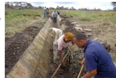
Farmers contribute to cleaning work of collapsed canal.
