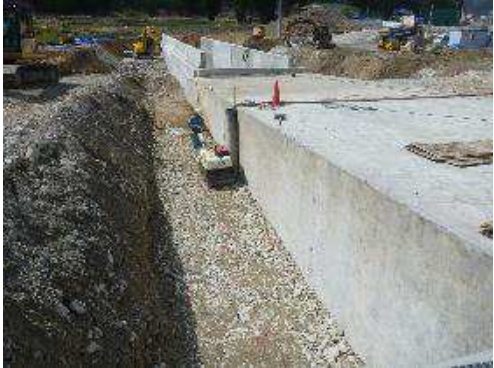
Backfilling at the culvert construction
