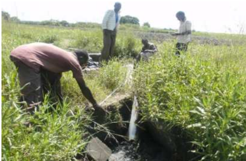
Vertical walls of the distribution boxes collapsed to the inside due to poor construction and abnormal earth pressure caused by black cotton soil.
