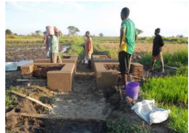
Farmers constructed division box using bricks.
