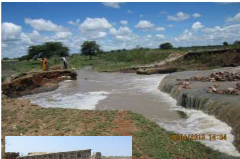
The scheme conveyance system was seriously destroyed by floods.
