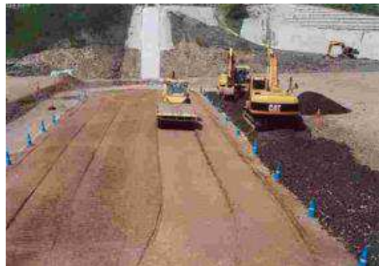
Compaction at the dam construction
