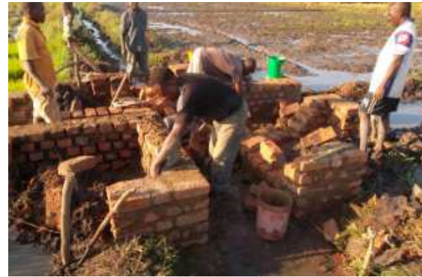
Farmers constructed division box using bricks.
