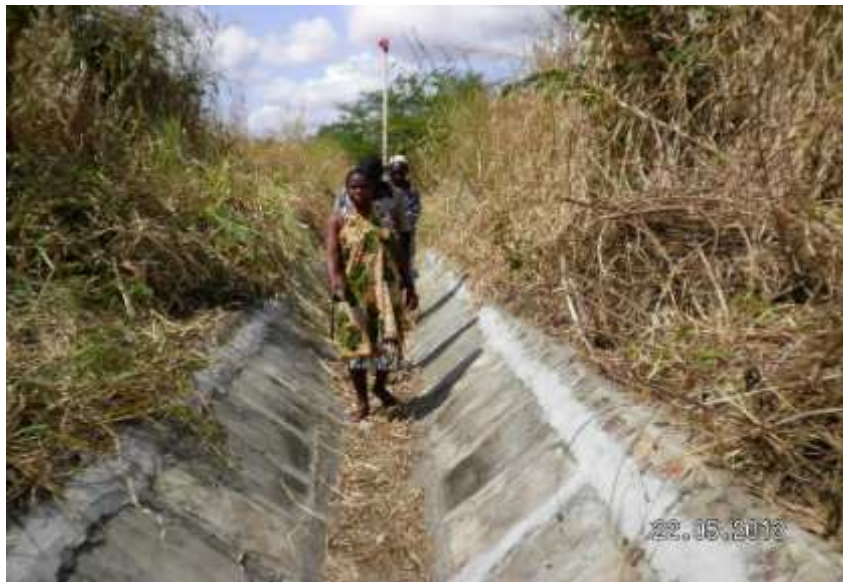
Some fields do not get irrigation water efficiently by differential settlement of the canal. Zone and District staff confirm the height of the canal bed and longitudinal slope.
