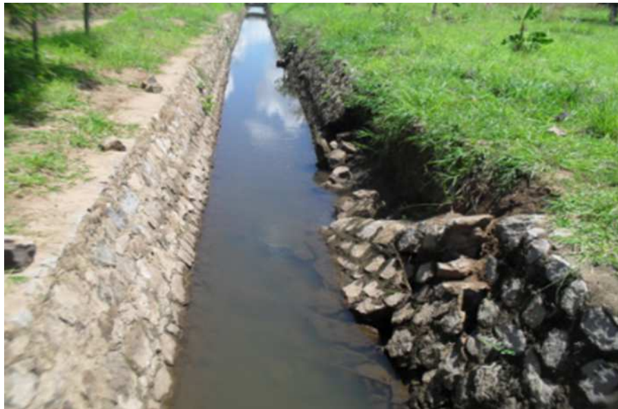
Side wall of main canal constructed by masonry collapsed. Some factors are picked up as the cause of this problem through the cause analysis.
