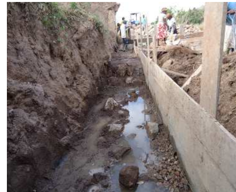
Increased depth of the embedment to 1.2m from the base of downstream apron.
