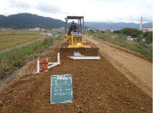
Banking at the road construction
