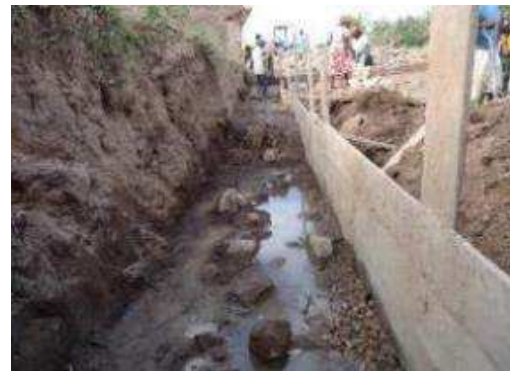
Embedment before concrete placement
