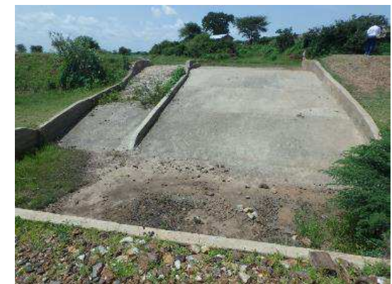
Additional spill way (right side) completed.
