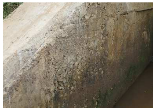
Cold joint caused by inadequate manner
