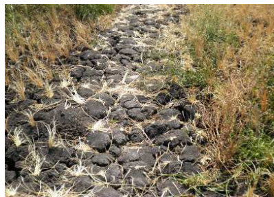
Cracked canal side wall caused by black cotton soil and poor compaction
