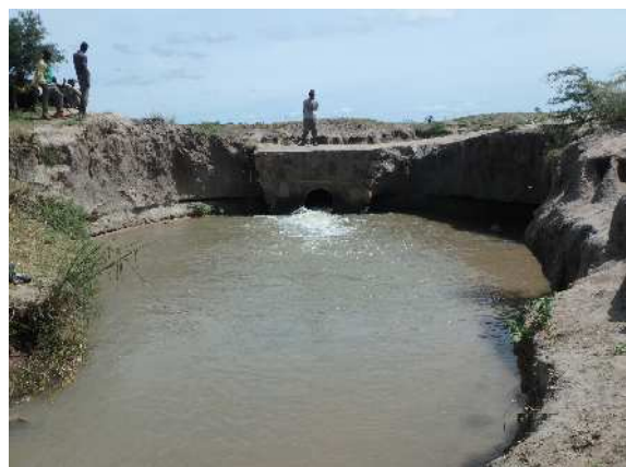
Scouring at the downstream of division structure
