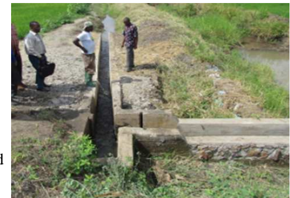
Rehabilitation work completed at the division box.
