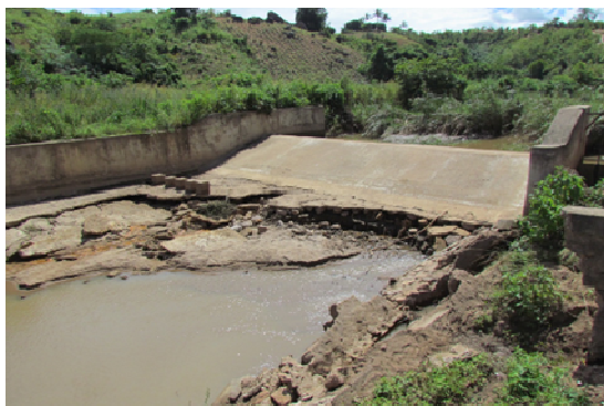
Base concrete washed away
