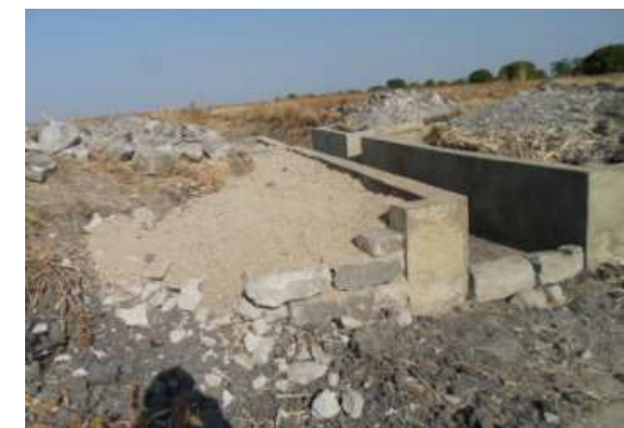
Compacted using crashed ole structure and morram beside the walls
