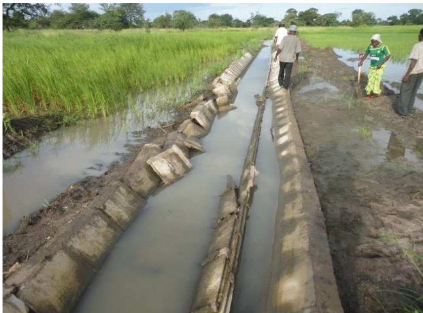
Bulging of main canal sides and cracks on slab joints caused by heavy rains with floods. (over-topping)
