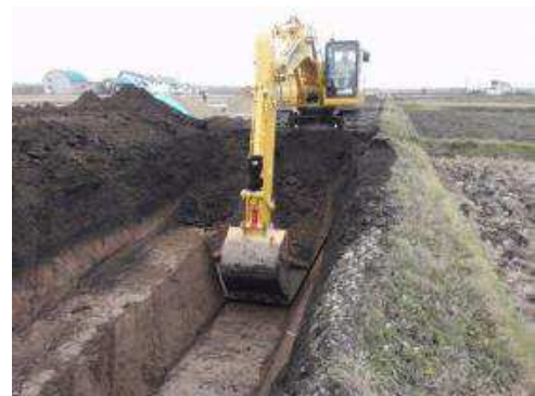
Excavation at the canal construction
