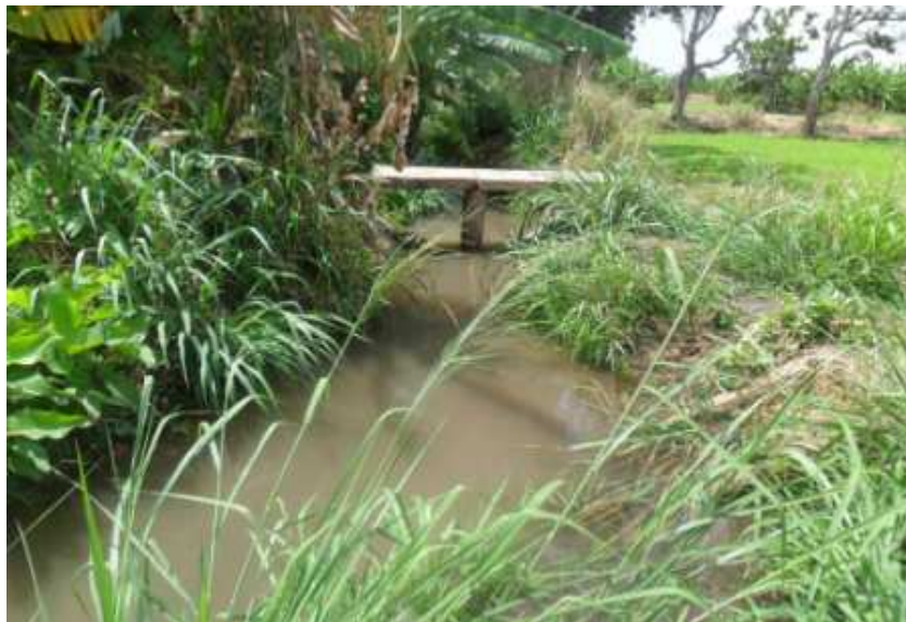
Since foot bridge was not protected from scouring, irrigation water was logging and seepage occurred.
