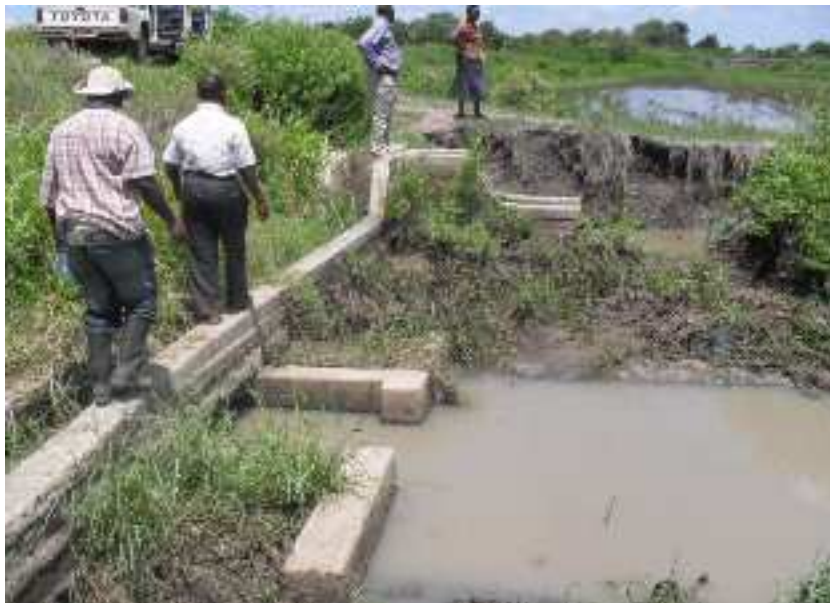
Secondary canal collapsed by flood water from adjacent pond. It was clarified that 5 Diversion boxes are out of order after Participatory Diagnostic Study.
