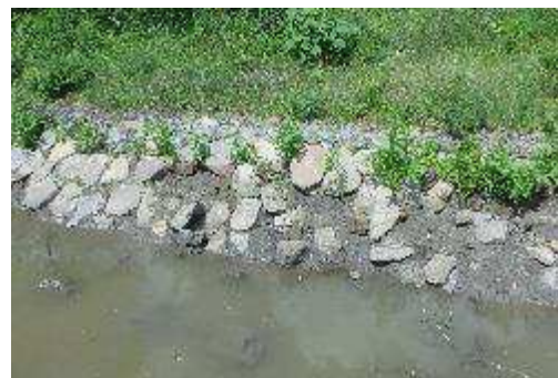
Deficit of masonry caused by washing out of backfilling
