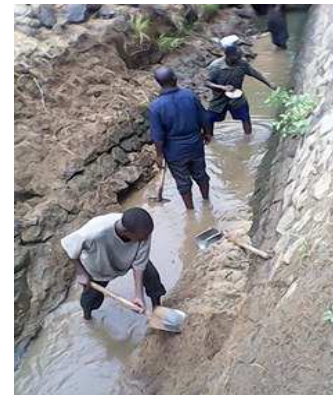
Construction work started from cleaning of sedimentation, and progressed with farmers' contribution
