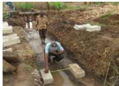
Construction works were pushed forward under supervision of technician.
