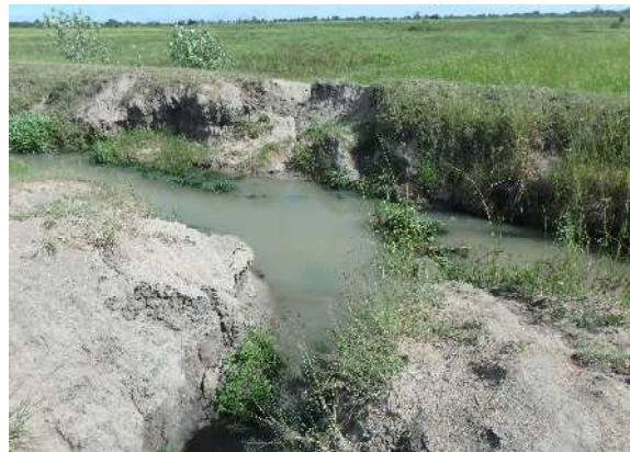
Erosion of side slope
