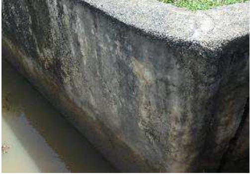
Hexagonal cracks caused by placing in high temperature condition
