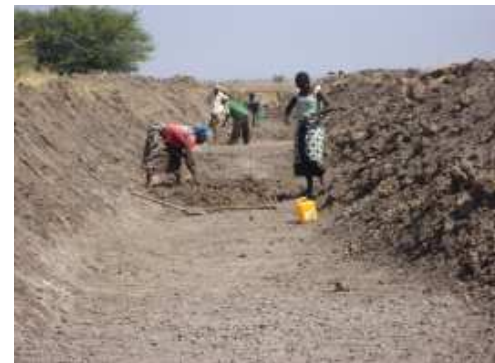
The main canal was widening by farmers' contribution.
