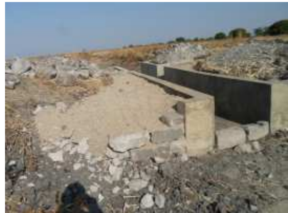
Concrete wreckage used as backfilling
