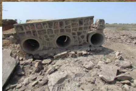
The scheme conveyance system was seriously destroyed by floods.
